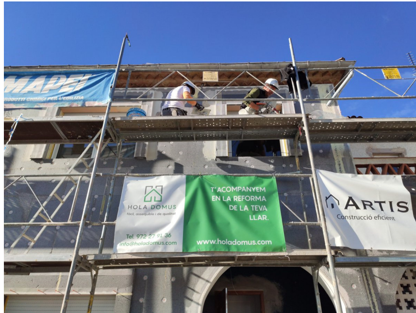
On-site works facade poster.
