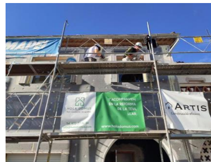
Figure 17 HolaDomus facade poster on construction site
